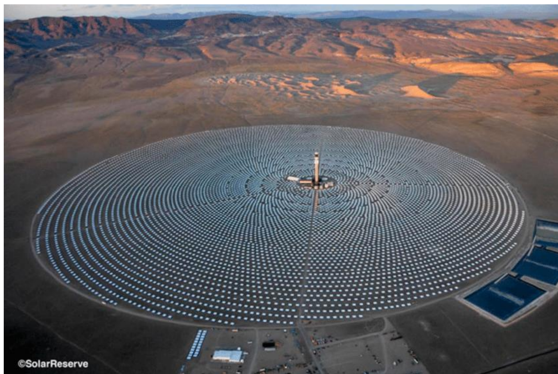
Crescent Dunes Plant in Tonopah Nevada contains over 10,000 heliostats
